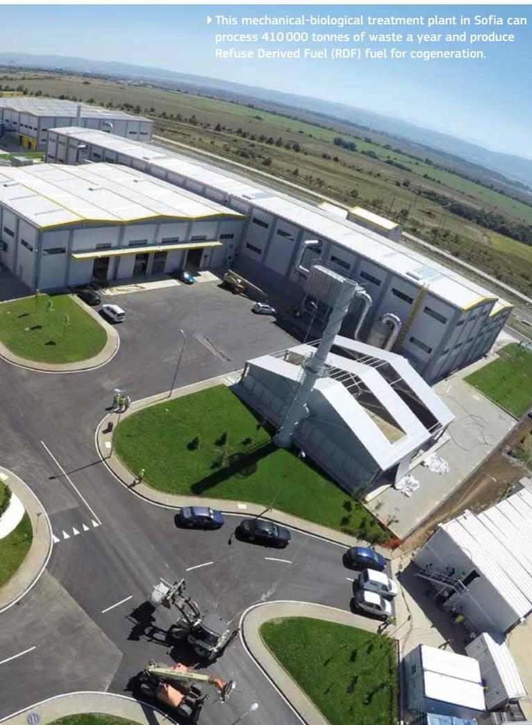
▶ This mechanical-biological treatment plant in Sofia can process 410 000 tonnes of waste a year and produce Refuse Derived Fuel (RDF) fuel for cogeneration.
